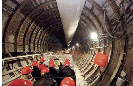
Workers riding tramway in Yucca Mountain access tunnel
